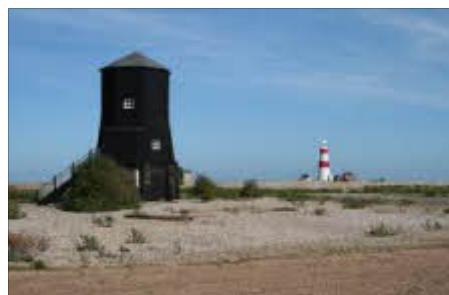
Beacon Navigation tower, Orford Ness
